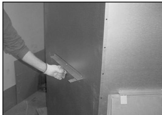
Figure 7.2 Bending Refractory Shipping Tabs Back Down
